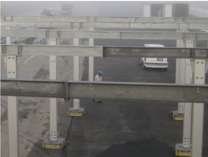
#8 Set second portion on top of uprights and bolt the rafters together at the end flange and then bolt the upright and rafter together.
