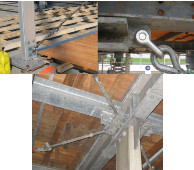
#10 After first bay of purlin beams are completed, install upright cables and lower roof cables.
