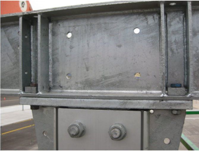
#7 Detail of upright to rafter connection.
