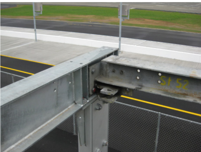
#9 Once two (2) arches are up, start at one end and install the "purlin" i-beams that run the length of the building. The larger of the two will be installed inline with the uprights with two (2) smaller beams in between. (Larger beam shown)
