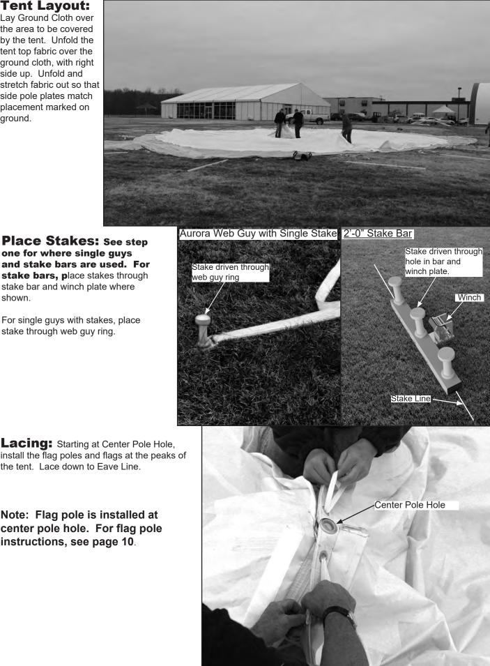
Lacing: Starting at Center Pole Hole, install the flag poles and flags at the peaks of the tent. Lace down to Eave Line.
